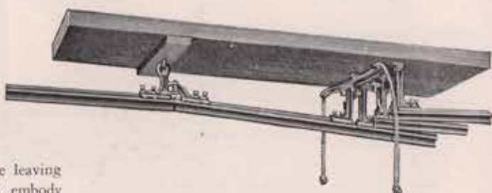
Fig. 805. Porter Three-Way Switch
