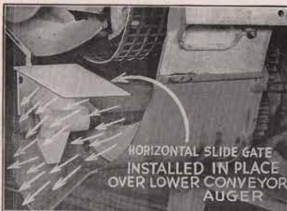
THIRD OPERATION ON ROUGHAGE Here the Preparation May End by Discharging the Chopped Roughage From Lower Conveyor Case, Or Continued, if Desired, By—
